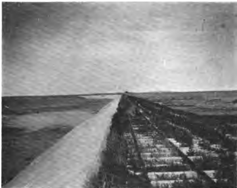
FIG. 201.—Owl Creek Dam, near Belle Fourche, South Dakota, Showing Concrete Paving.
